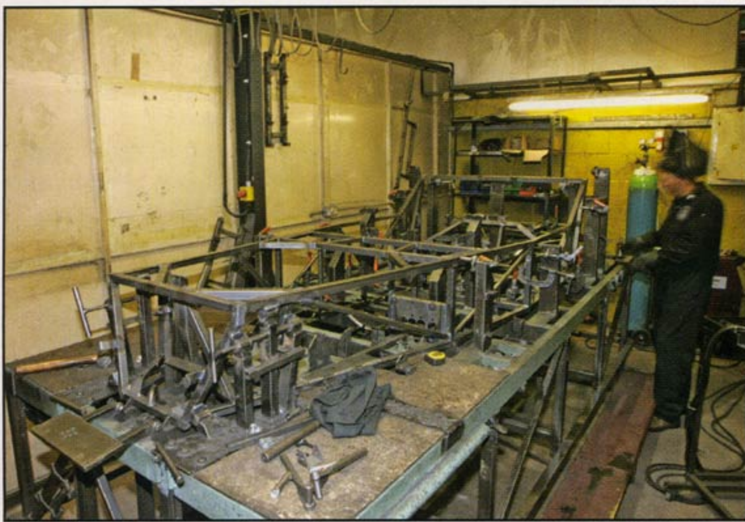
The chassis are welded up in these jigs for precision alignment.
